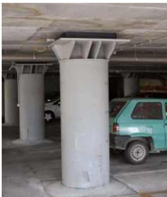
Figure 6. Base-isolation of a residential building in L'Aquila, Italy (courtesy of D. Pohoryles)
